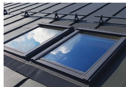
Bar-type snow guards fastening detail
